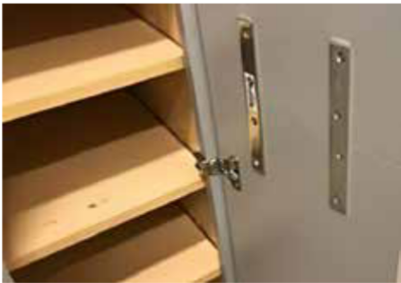
Interior of door with metal brackets
